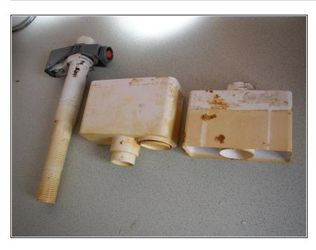
Here you can see the parts of the valve. The seal is the red dot!
