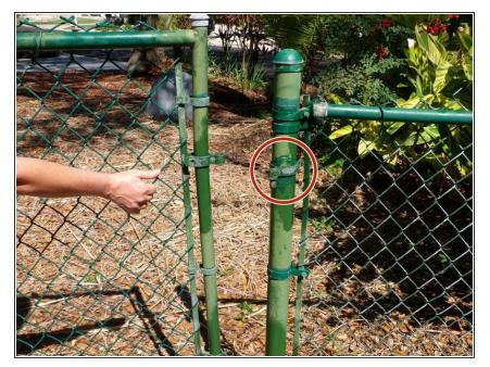
• Remove the unbolted post hinges from the fence posts.
