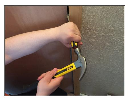
Take the hammer and hit the handle end of the screwdriver until the pin can be pulled out. This may take a while depending on the door.
