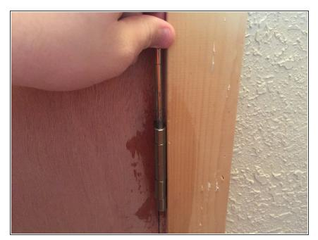
Take the pin from the bowl and reinsert it into the door hinge, using a hammer if necessary.
