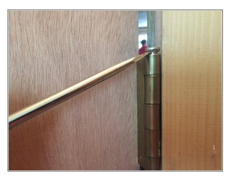
Insert the end of the flathead screwdriver into the crease between the top of the pin and the hinge.
