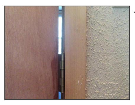
Open and close the door a few times. This will help the oil to seep into the cracks of the hinge.
