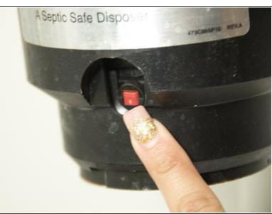
Press the red reset button either on the front or on the bottom of your garbage disposal.
