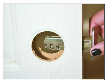
• Slide the latch of the deadbolt back into the door frame.
