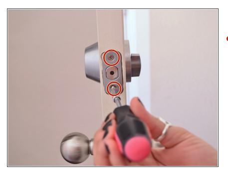
Use a Phillips screwdriver to screw in both of the <sup>3</sup>/<sub>4</sub>-inch screws back into the strike plate.
