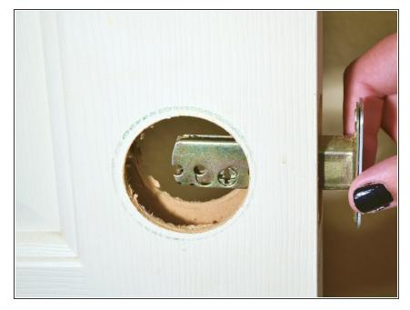
• After all four screws have been taken out, slide the latch of the deadbolt out of the door frame.
