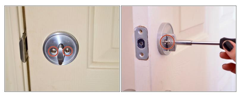
Remove both of the 2.5 inch mounting screws from the lock cylinder.
