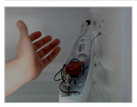
Replace the old thermostat and reassemble the new thermostat using the picture that you took before to properly connect the wires.
