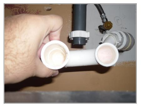
Clear out the gunk, obstructions, and any other objects in the pipe so that your sink drains properly.
