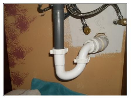
When you first go to clear your sink, you should check how the pipes are connected.
