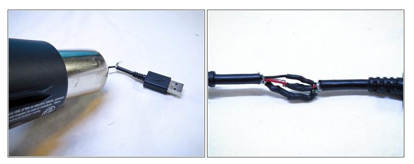
• Next you can use a heat gun to melt the heat shrinks together for maximum wire protection.
