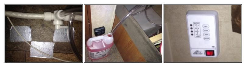
A The installation of a Tee was necessary so as not to have to dismantle the connector from the tank
