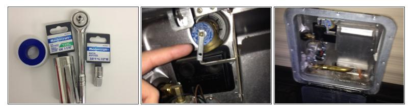
• To drain the water heater, the anode must be unscrewed with a 1 and 1/16 inch socket.
