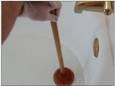
Without breaking the seal of the plunger on the drain, push the plunger sharply down and up a few times.
