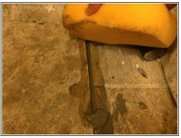
After leveling the tiled area, use a damp sponge to remove any excess mortar that may be on the tile.
