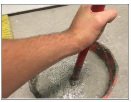
The first step is mixing your thin-set mortar and water into the five gallon bucket. (Precise ratio will be on mortar packaging)
