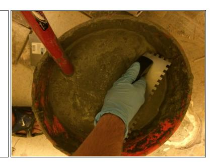
Once you have spread the amount of mortar that you will need, use the trowel once more to clean the excess mortar from the floor. Excess mortar can be returned to the bucket.
