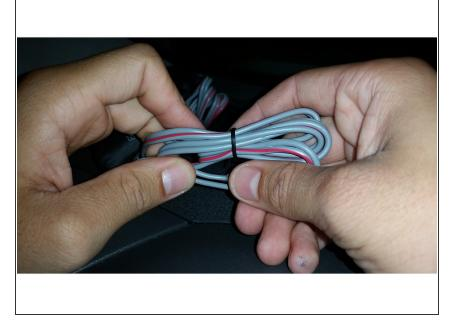
Take any excess cable and fold it neatly so that it will fit down the hole below the tweeter.
