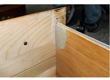
Apply the wood putty to the freshly sanded corners. Smooth the wood putty evenly, applying moderate pressure to ensure stable reinforcement.
