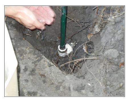
Clean the area around the fitting with water until the fitting is mostly free of dirt.
