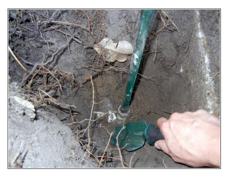
Dig around the pipe fitting with a trowel to provide clear access.
