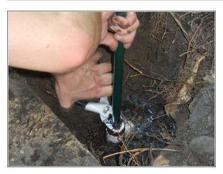
Screw the new sprinkler extension in securely.
