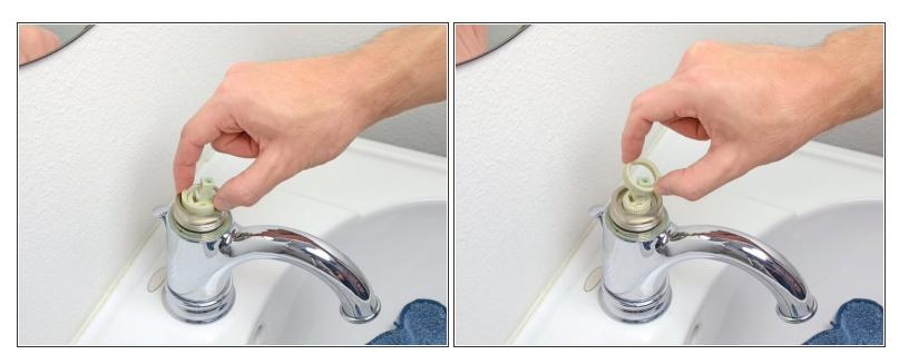
Remove the temperature limit indexer from the top of the cartridge.
