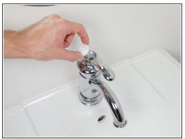
Use your fingers or a prying tool to remove the plug button from the top of the faucet handle.
