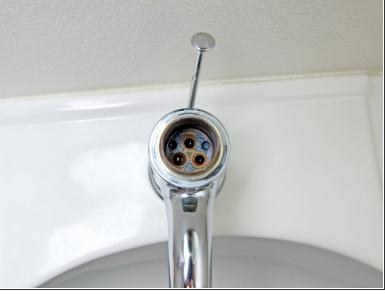
When reinserting the cartridge, be sure that the keys on the cartridge line up with the keys on the base of the faucet.
