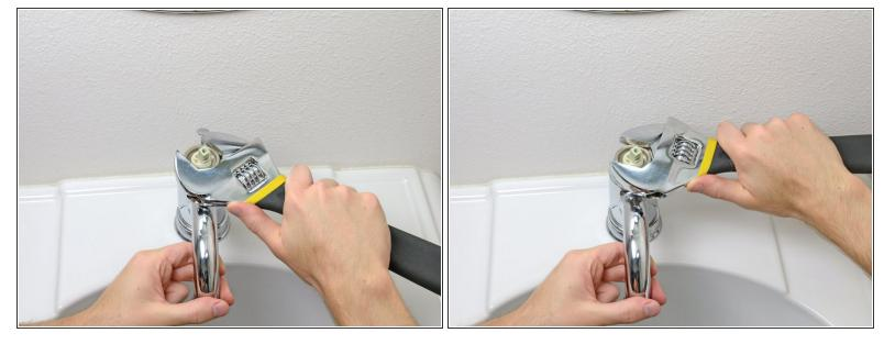
Use an adjustable wrench to loosen the bonnet nut.
