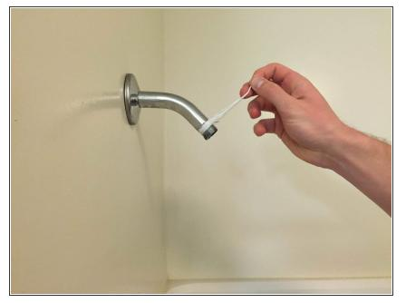
Remove the old plumbing tape from the threads of the pipe, and throw it away.
