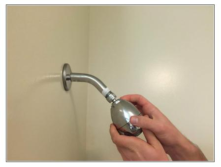
• Begin installing the new shower head by threading it onto the pipe.
