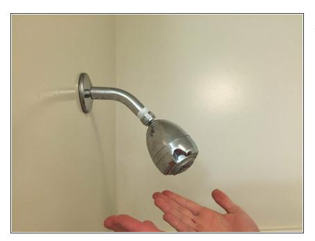
Use your hands to tighten the new shower head back onto the pipe, using a wrench if needed.
