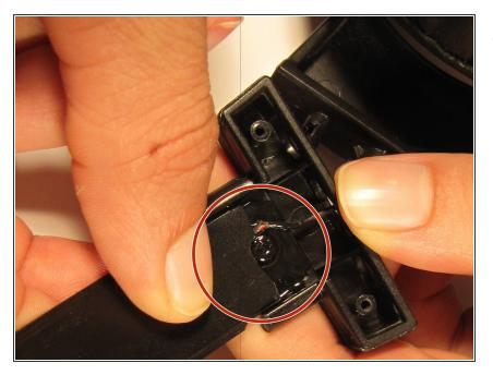
Clamp the pieces in place by hand or with a binder clip until the Plasti Dip dries. Feel free to use a hair dryer on a low setting to speed up the process.
