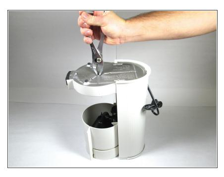
Locate the nut at the center of the base and unscrew it with a pair of basic pliers.
