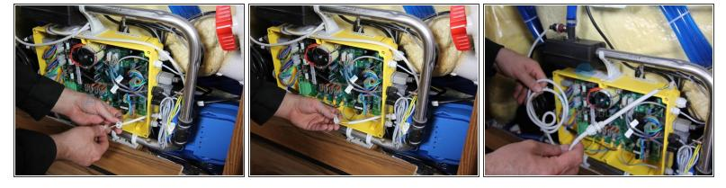
Route the pressure switch cable out of the control box
