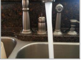
Turn on water and check for leaks at faucet and spout
