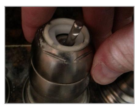
Hand tighten plus a little turn with channel lock pliers. Do not over tighten or scratch finish.
