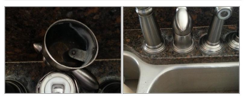
Insert ball stem into hole in faucet handle and tighten set screw
