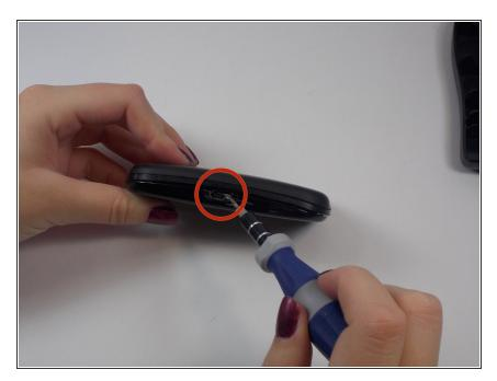
Turn phone over on its left side and remove single phillip's head screw using the Phillips #0 screwdriver.
