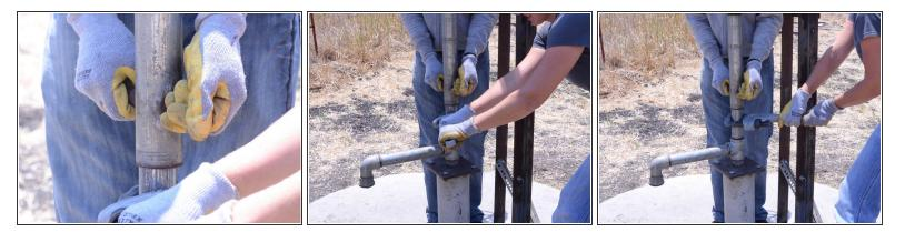
• Use a pipe wrench to fully loosen the above grade riser pipe.
