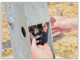
Remove the nut from the chain bolt.
