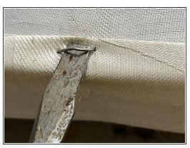
Lift the staples with the flathead screwdriver before going in with the pliers.
