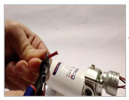
Use the cutting plier or (if you have it) the stripping plier to remove the sheath.
