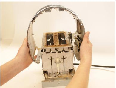
• Lift up the part of the handle together with the top cover of the toaster.
