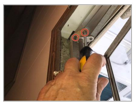
Using a Phillips screwdriver, remove the two screws from the mount at the opposite end of the bar.
