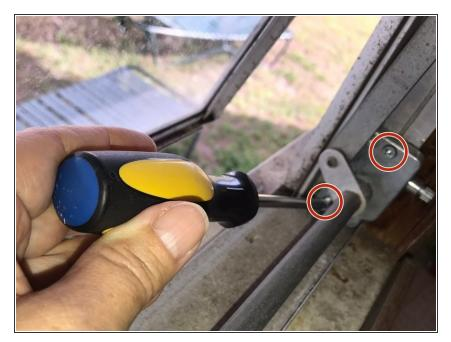
• Using a Phillips screwdriver, remove the two screws from the gearbox.
