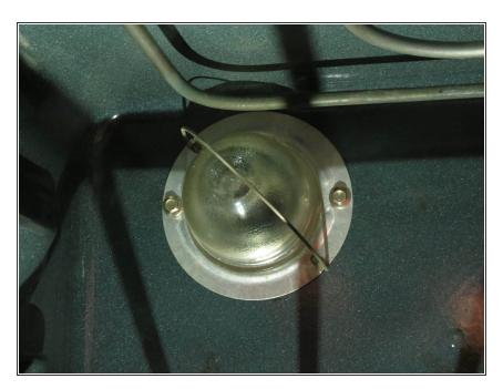
Locate the metal strap holding the glass cover over the bulb.
