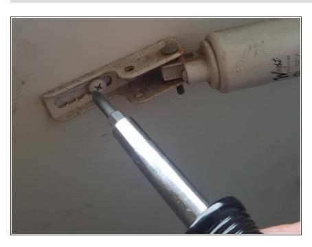
Loosen the screws from the bracket on the screen door to remove the bracket.
