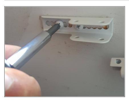
Install new bracket onto screen door. Keep screws slightly loose.
