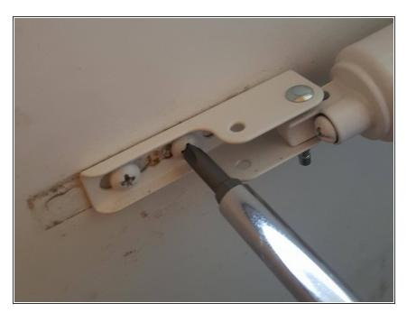
Slide the bracket away from the barrel until there is no slack. Tighten screws on the bracket.
