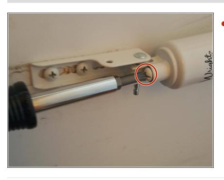
Test the door and if there are any issues (i.e. door closing too fast or too slow). Make necessary adjustments to the tension screw.
