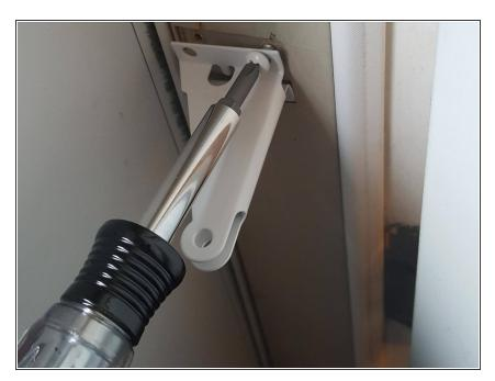
Attach the new bracket to the door jamb with provided screws.
