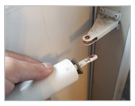
After removing the pin, the closer barrel can be removed.
